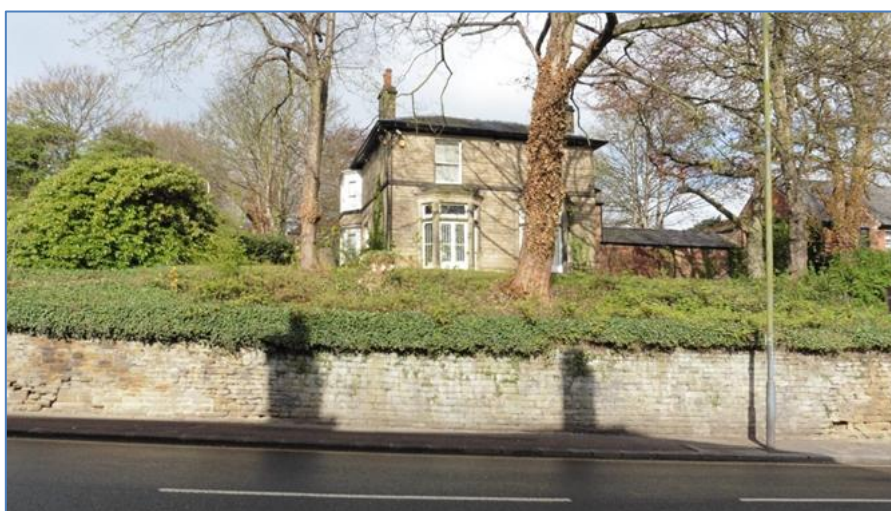
Figure 1. Ashton Lodge - Sheffield Road elevation
